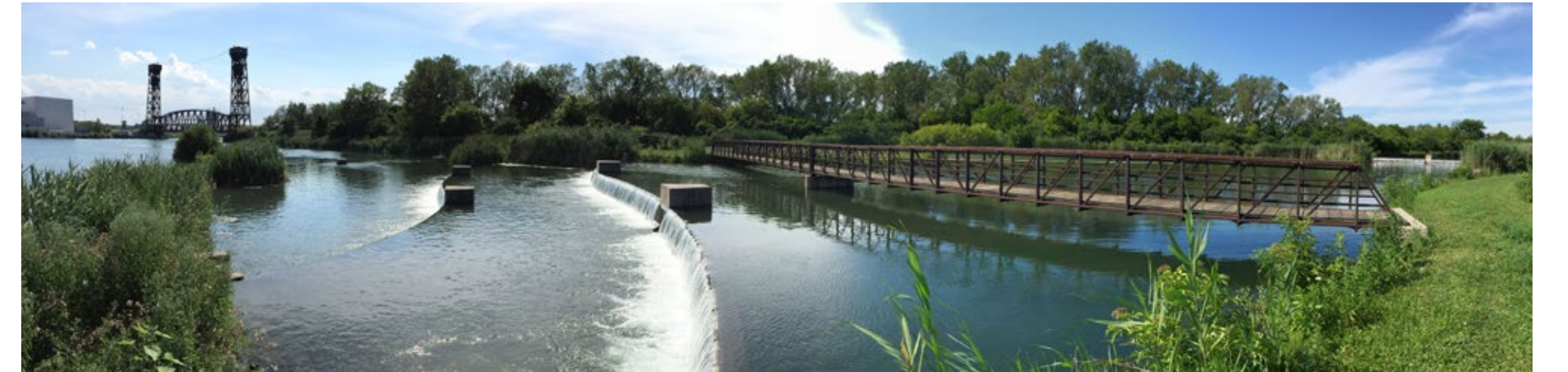
Sidestream elevated pool aeration stations, like this one on the Calumet River, are an attractive way to reduce odor and improve water quality.
