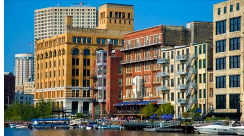
Formerly industrial buildings along the Milwaukee River now contain homes and businesses with river access.
